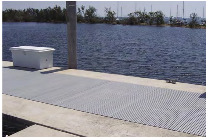
Strongwell's DURAGRID® T-1700 pultruded grating was used to replace wood planks on a large walkway at Dinner Key Marina in Miami, Florida. The grating allows for easy accessibility to utilities below the walkway and will not rot like the previous wooden walkway.
