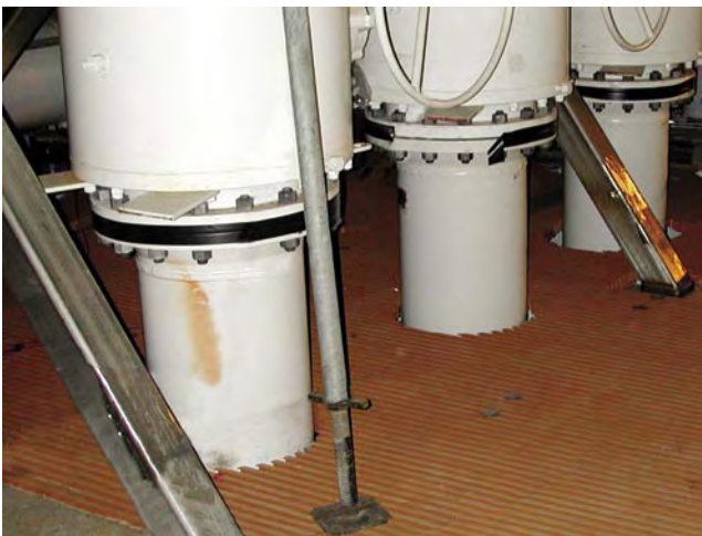
DURAGRID® Phenolic Grating's unique construction allows for many penetrations to be cut without adding additional supports.
