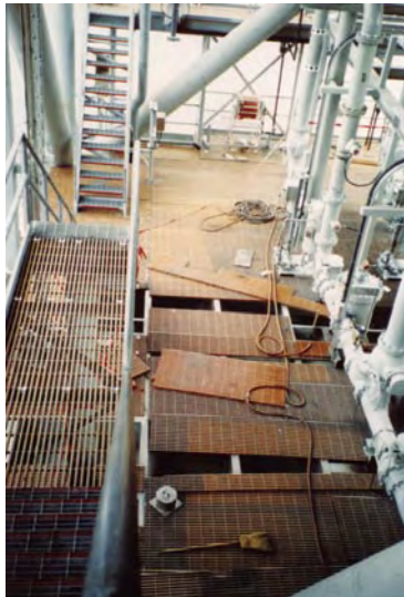
DURAGRID® Phenolic Grating's unique construction allows for many penetrations to be cut without adding additional supports.
