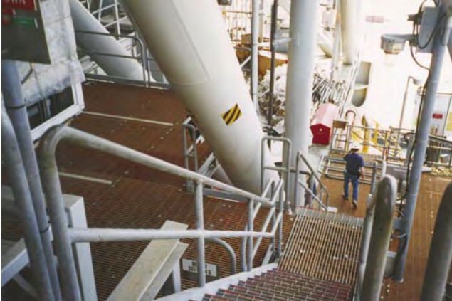
DURAGRID® Phenolic Grating has been used to reduce weight and maintenance on offshore oil production platforms for more than a decade.
